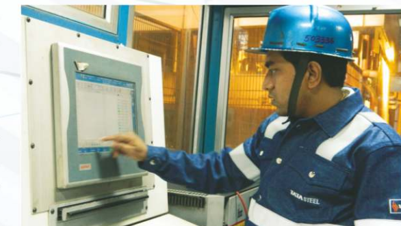
Control Room for On-line Non Destructive Testing
