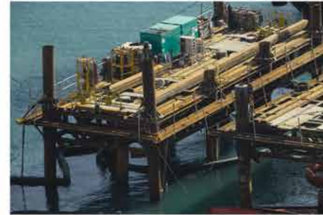
Tin Tunnel project
