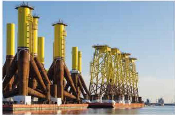
Foundation for wind wheel
