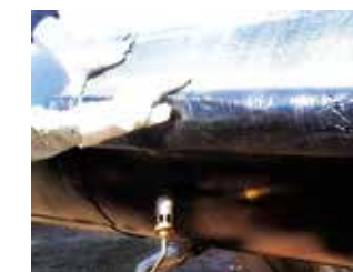
Coal Tar Tape Application
