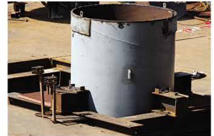
Steel pipe pile foundation for bridge construction
