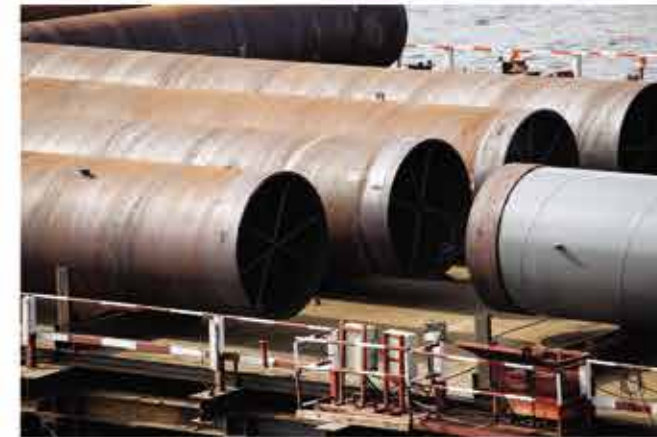
Steel pipe pile foundation for bridge construction
