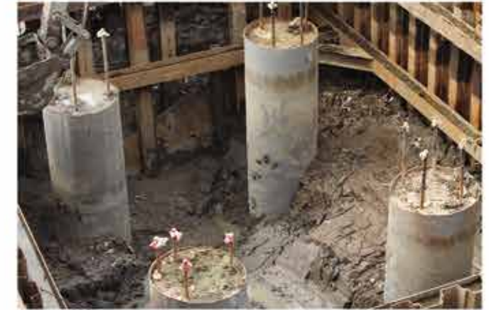
Boring pile for bridge foundation
